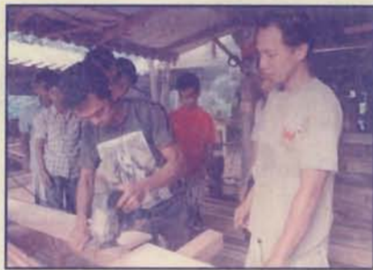
1. Choose wood to be perforated at eaves (soft wood should be chosen)
