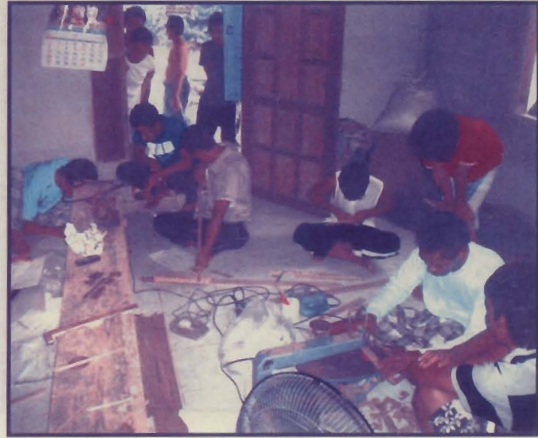
4. Make pile of bird's cage under design
